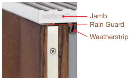
Top of door; exterior view.
